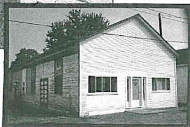
The ubiquitous "cove" pattern, also called "novelty" in its own right. Cove siding was popular by 1880, and may have been patented fifteen years earlier.
