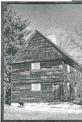
Buttolph Williams House, Wettersfield, Conn. (1692). Skived clapboard, 3 3/4-inch exposure.
